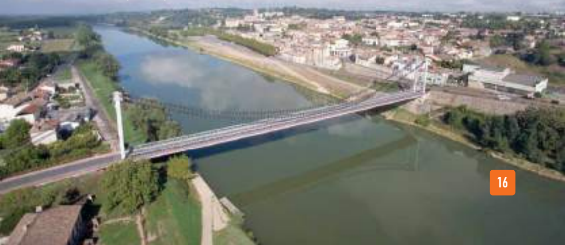
View from Rouergue bridge
