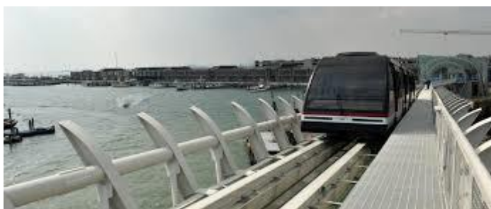
Figure 53 The 'people mover': an elevated infrastructure for public transport of people (source: SEAP of the Municipality of Venice)
