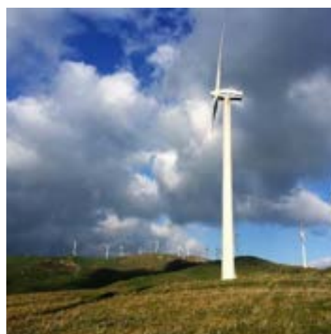
Figure 51 The wind energy plant, built in the area at the beginning of 2000
