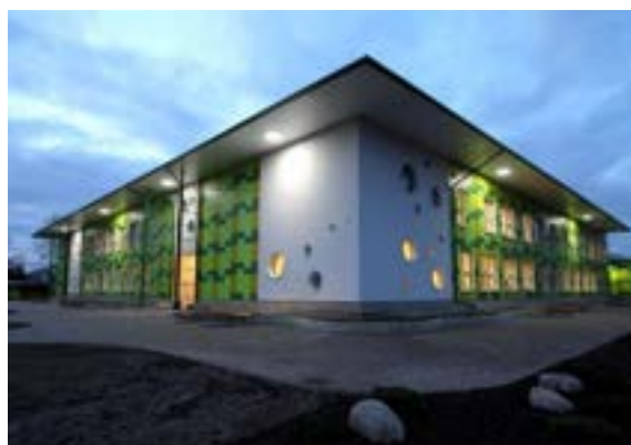
Figure 30 Rakvere Rohuaia Kindergarten, Source: http://www.te.ee/est/objektid/2015/rakvere-rohuaia-lasteaia-ehitustood
